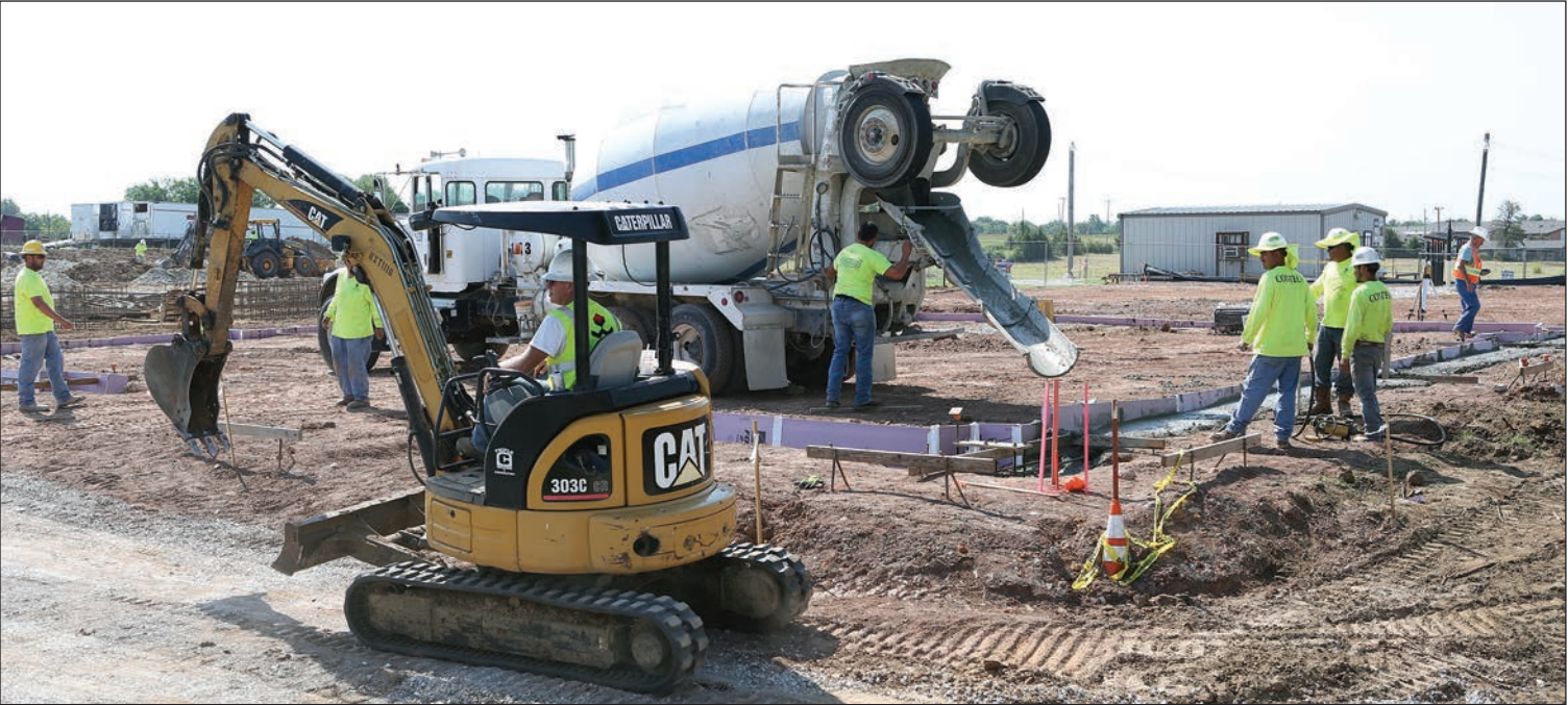
Work crews are pictured pouring reinforced concrete footings to support the foundation on the new facility being constructed in Stroud for the Sac and Fox Na-
